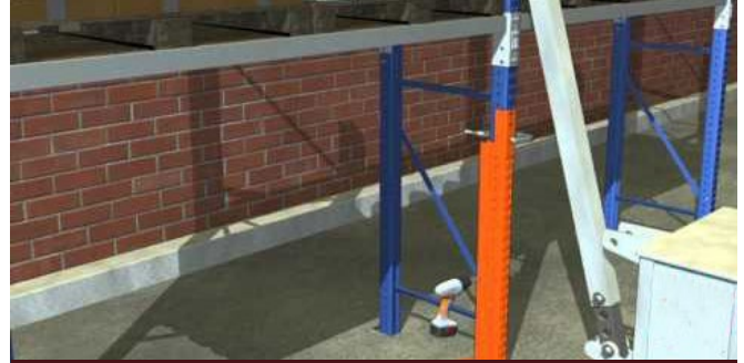
Prep & Cut Out Damage
